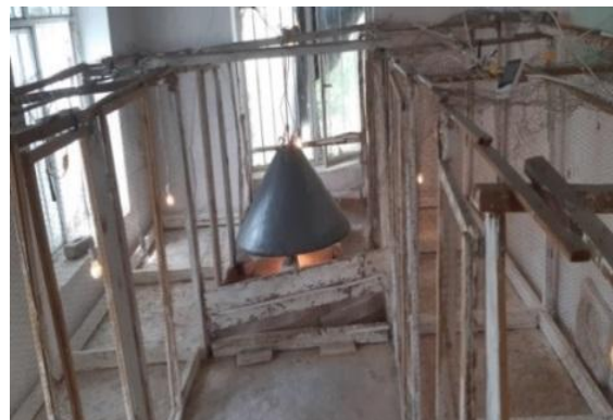
Figure 2. Interior View of the Poultry House
